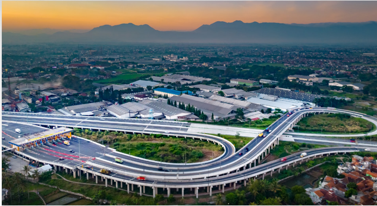
Highway in Indonesia connecting mountains with industrial zones.
